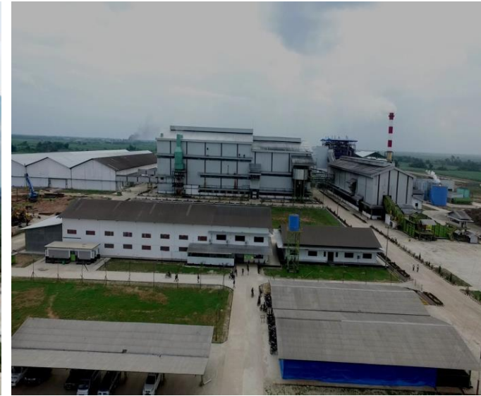
SUGAR MILL – Capacity 8,000 TCD (Ton Cane Day), or \pm 100,000 ton/pa of sugar
